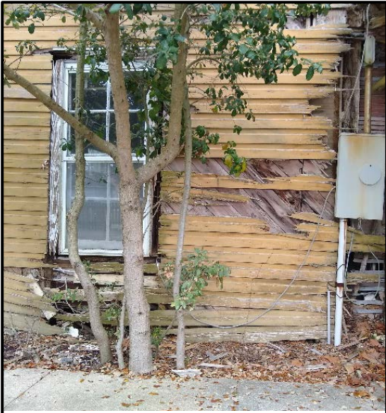
Example of the condition of the exterior siding and deterioration at sills
